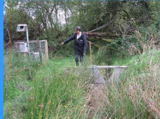
Monitoring equipment at Boldventure
